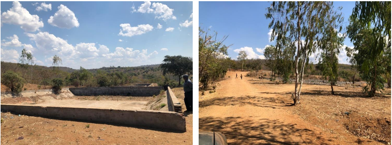
Figure 5.19: Incomplete liquid containment ponds and unsecure waste disposal site (Sosola)
